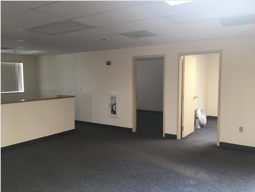
Knee wall area outside of 11' by 18' private office
